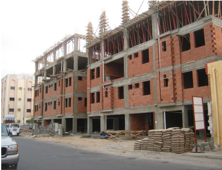
Figure 1: Simultaneous construction of 2 residential apartments inside the city.
